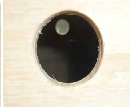
Figure 8: Close up of top (open) ventilation holes (K. Elliott, 2009).
