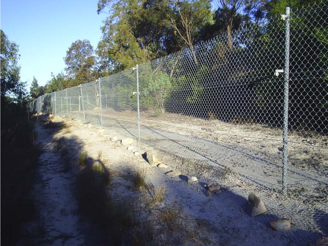
Figure 1. Electrified feral predator-proof perimeter fence at Australia Walkabout Wildlife Park (Photo: N. Carson).
